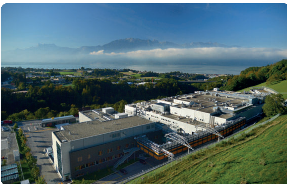
Merck biotech development center in Corsier-sur-Vevey EURO 250M investment
